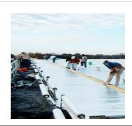
Sky Web II Fall Protection and Insulation Support System-The Sky-Web-II® System is an innovative passive restraint system that protects workers from falls at the leading edge of a roof. It provides a "web" of knotted nylon mesh that is attached to the perimeter of the roof's secondary structural members. This products leads to an increase in safety and reduces injury
