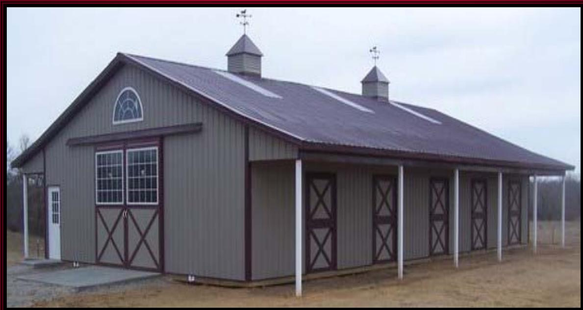
MBS Self-Storage buildings offer a wide variety of layouts– Typically based on 5ft spacing. Common roof slopes 1:12 to 1/2:12 and eave heights of 8'6 or 9'6 . All roof and wall panels are made from strong 26ga sheeting either bare galvalume or painted sheeting with a 45 year warranty. Interior partition panels commonly use 29ga bare galvalume
