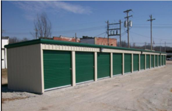
Steel Building kits from Metal Building Supply offer many advantages you won't find in other buildings. All building components are pre-cut, pre-punched and ready to bolt together in the field w/ solid I-beam frames all engineered for your area. You will receive a comprehensive set of erection drawings showing all details. All buildings are made with the highest quality Materials, all painted sheeting carries a 45 year warranty.
